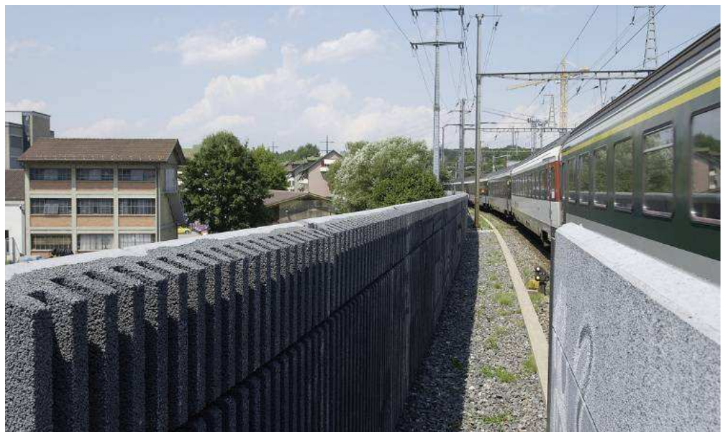
Figure 8 – Noise Barrier in Switzerland
