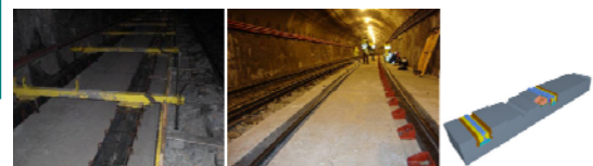
REMS installation in a tunnel of the Madrid metro network
